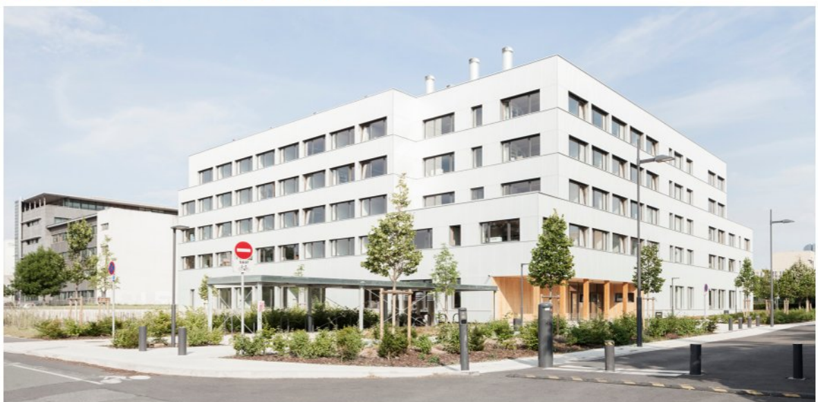
© Schnepf Renou photographe © Atelier Pascal Gontier
